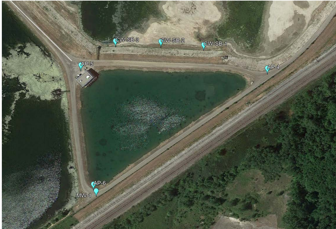
Figure 7. Approximate Boring/Monitoring Well Locations at Clear Water Pond
