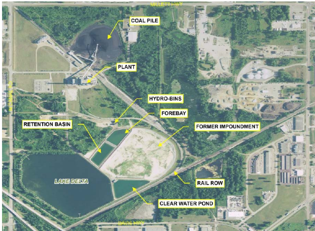
Figure 2. Erickson Power Station Site Configuration
