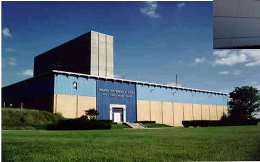
Wise Rd. Water Plant - 1966
