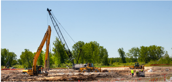
Construction work at Delta Energy Park.
