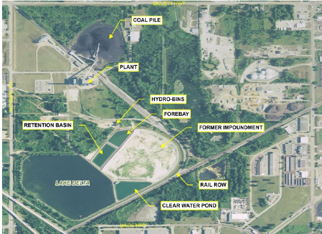
Figure 2. Erickson Power Station Site Configuration
